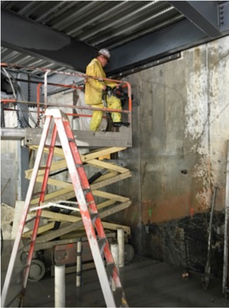
Opening the concrete wall under the kitchen
